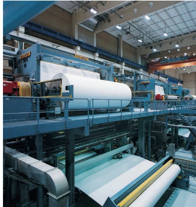
High level of availability of the Motor Control Center even in a harsh industrial environment
