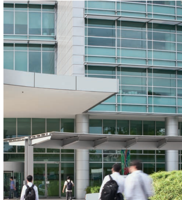
In office complexes, space-saving and cost-effective switchboard installation is requested.
